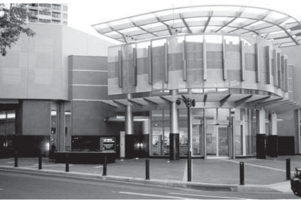
Entrance to Brisbane Arrest Courts at 240 Roma Street, Brisbane
