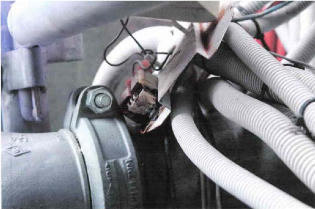
Photo taken by Garaty shows inners of light resting on scaffold
