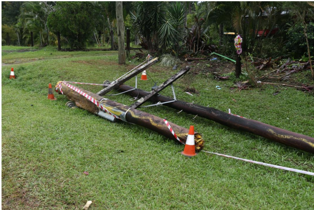
Power pole sheared off through impact
