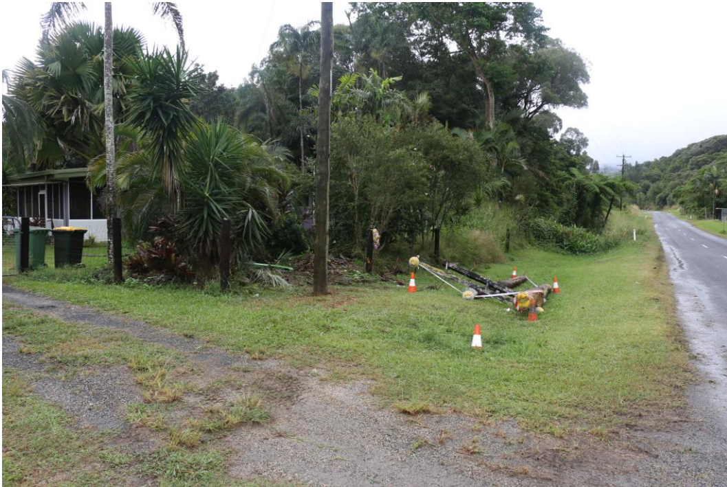
Replacement power pole in position
