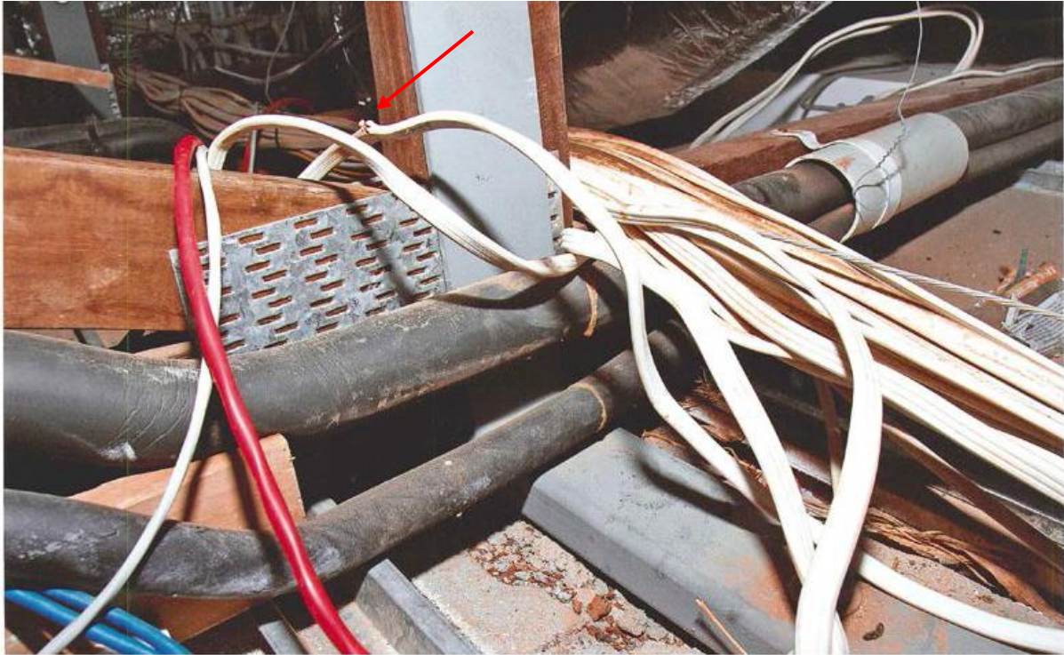
Photograph depicting circuit 22 cable positioned above the gang nail plate
